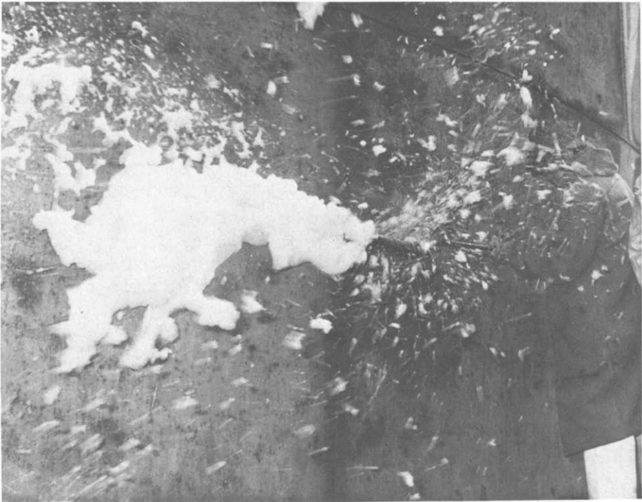
Fig. 9. Hot cutting showing foam purging.
